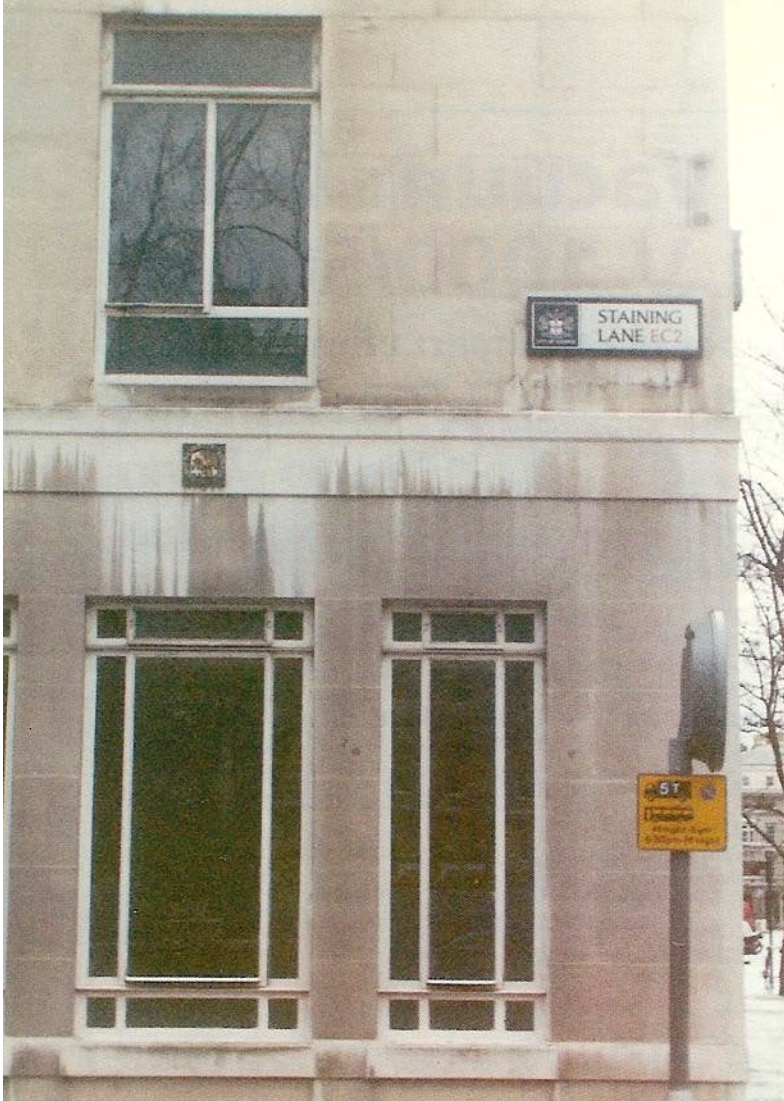
Lime runs on stone discoloured by the effects of long term pollution.
