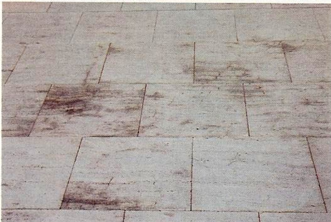
Left: Fig 4. Dark patches in a travertine floor due to different concentrations of dirt in unfilled voids. Above. Fig 5. Discolouration of Carrara marble.
