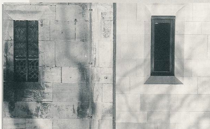
Above. The original, 700-year-old building of York Minster and the new extension. The difference is stark now, but the new Cadeby limestone will quickly weather to match the older stonework.
