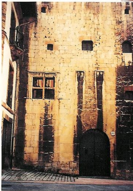
Above. Tower of the Cathedral of Oviedo in north-west Spain. It was mainly built using a medium density limestone. A black crust developed as a result of pollution.
